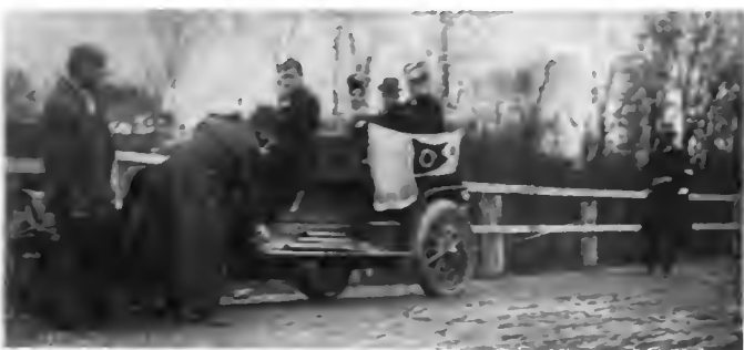
CLUB SURVEYORS CHECKING MUSKOVIC'S FRAYER-MILLER.
